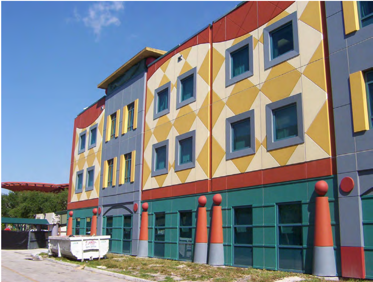
Fig. 14 Miami Hospital clad in hurricane resistant GFRP panels
